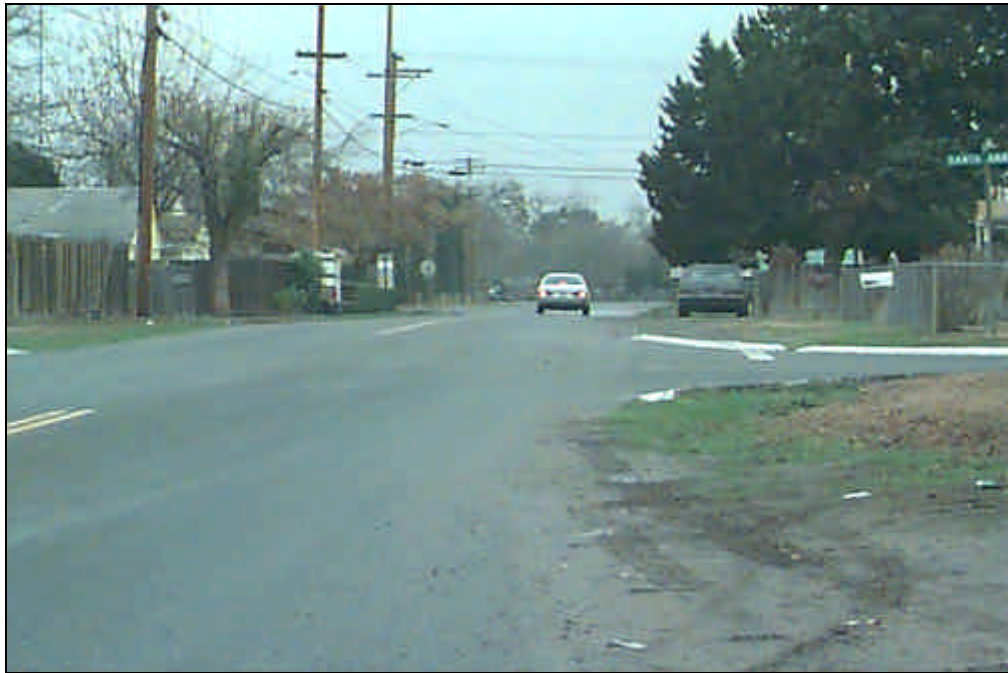
Figure 19: Tenaya Road at Santa Ana Avenue without Curb, Gutter and Sidewalk
